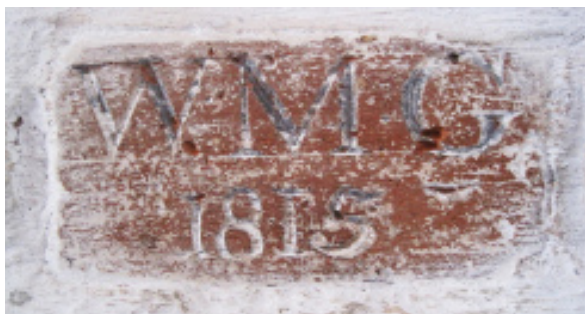
Architects sometimes sign their buildings. Lieutenant William Matthew Gossett was Commanding Engineer at York when he caused his initials and the year to be carved into a brick arch in the interior of the Stone Magazine. Photo by Chris Laverton
