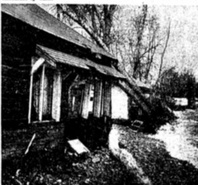
View looking out from 185 Lake Promenade shows wrecked house, was erosion.
